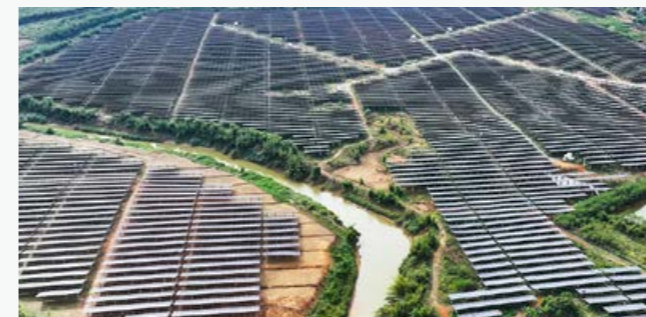
Survey Site of Photovoltaic Green Supply Chain Action
